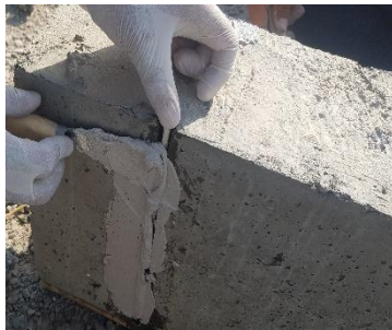
The GFRP bar was glued by sikadur-3
