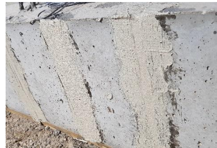
d. Finishing beam surface
