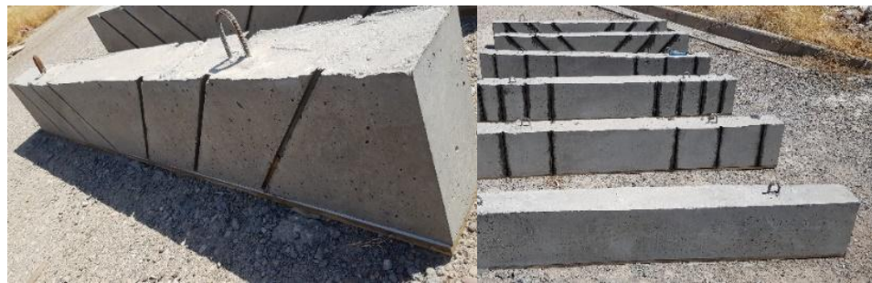
a. Making the grooves
